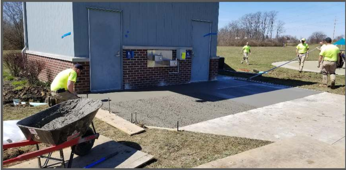
Team Members replaced a concrete panel at Flagship Park.
