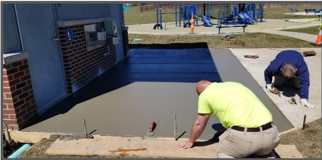
Team Members replaced a concrete panel at Flagship Park.
