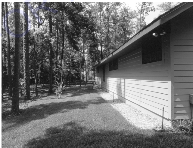
FIGURE A.17.1.6.5 Mitigating Risk of Leaf- and Needle-Filled Gutters. [1144: Figure A.4.2.2.5]
