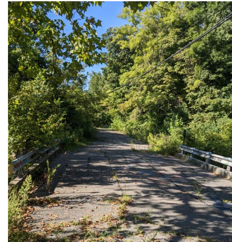
3. The bridge where the creek forks join together
