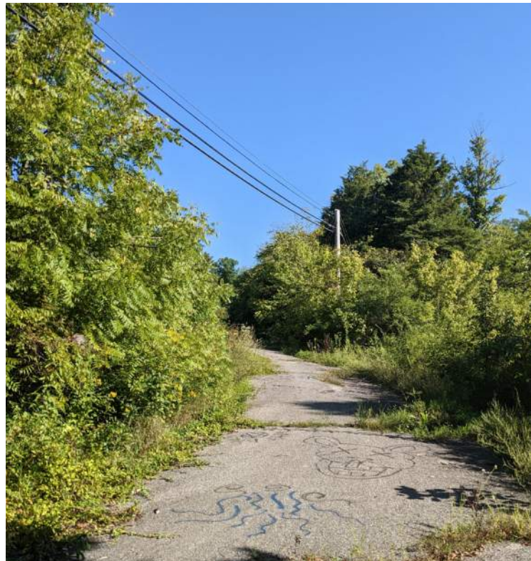
1. Looking north up toward Turfway Road
