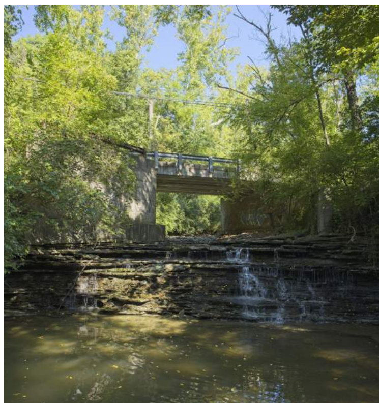
5. In the creek; looking underneath the bridge from image 3
